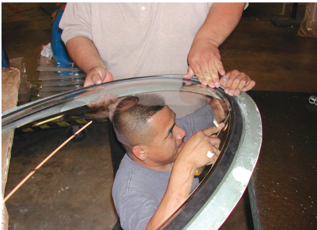
Photo 28 Installing the mock-up acrylic window in a mock-up fiberglass frame made by Mr. Donaldson at Planet Plastics, Corona, CA, May 22, 2003, Milford Wayne Donaldson, FAIA, photographer.
