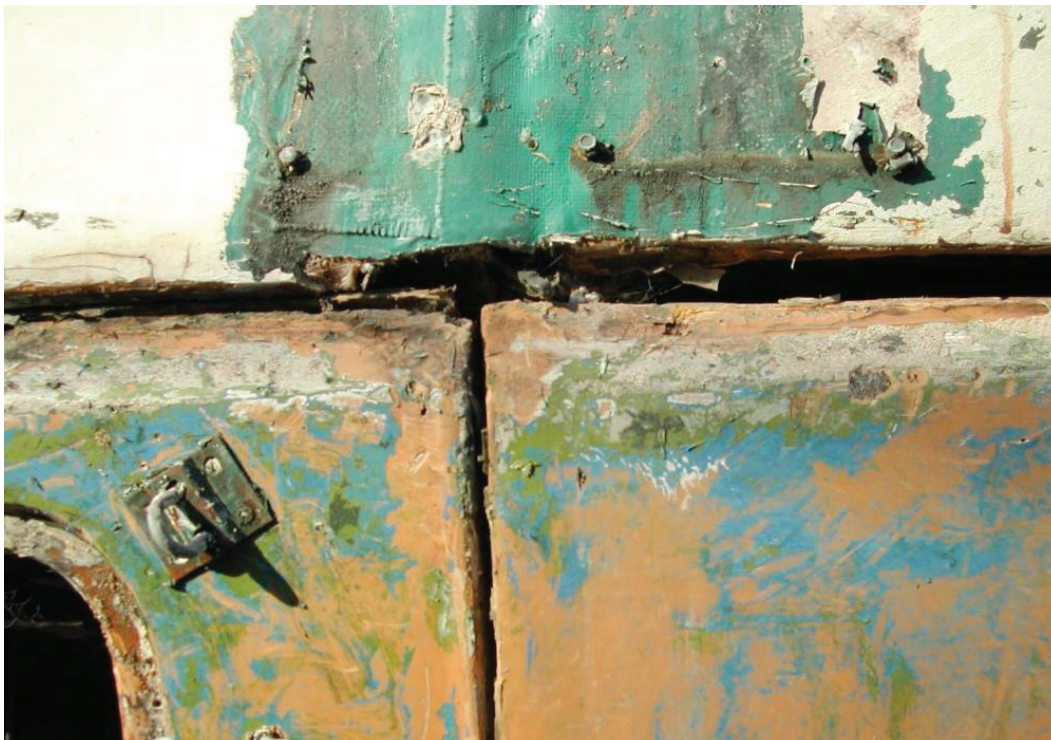
Photo 27 Near top of door opening where upper and lower halves of shell are joined; vertical joint is connected with steel bolts from the bottom but the top was fiberglassed together in one piece. December 2002, Milford Wayne Donaldson, FAIA, photographer.
