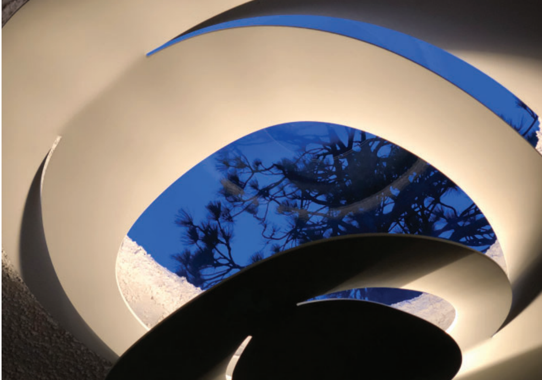
Photo 9 Restored opening for central fireplace, adapted for acrylic skylight and light fixture, n.d. Milford Wayne Donaldson, FAIA, photographer.
