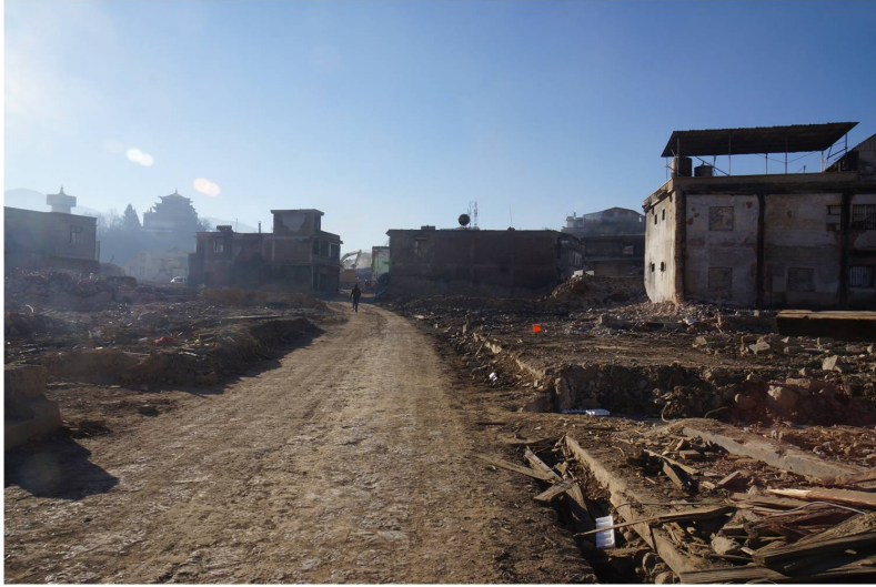
Figure 2: The same street after the 2014 fire
