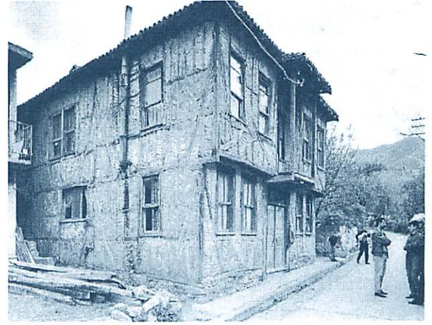
Gölcük, This 2-story house in traditional Turkish construction dating from the early 20th Century survived the Kocaeli Earthquake, undamaged, one block away from many modern reinforced concrete buildings that completely collapsed.
