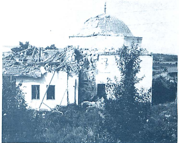
Rogovo, Kosovo — Mosque of Kel Hasan Aga, built 1580. In May 1999, Serb police and paramilitaries packed the interior staircase of the minaret with explosives and blew it up, causing the tall spire to collapse onto the dome and roof of the mosque. Remains of the base of the minaret can be seen to the left of the domed main prayer hall. (Photo: October 1999, Andrew Herscher, Kosovo Cultural Heritage Project, Harvard University)
