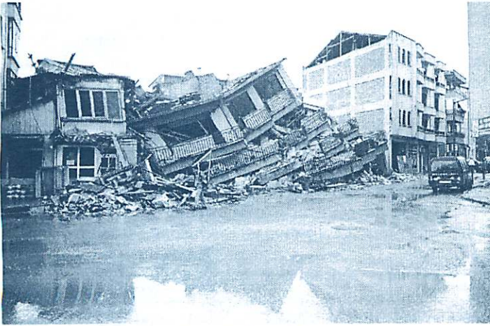
Collapsed multi-story apartment building, Adapazzari Like thousands of other buildings in this city and others near it, this building collapsed. Over 25,000 people died in collapsed reinforced concrete buildings
