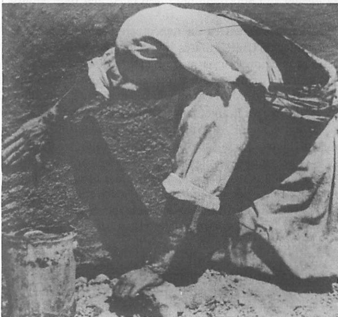
Traditional manner of applying mud plaster. Photo courtesy Museum of New Mexico
