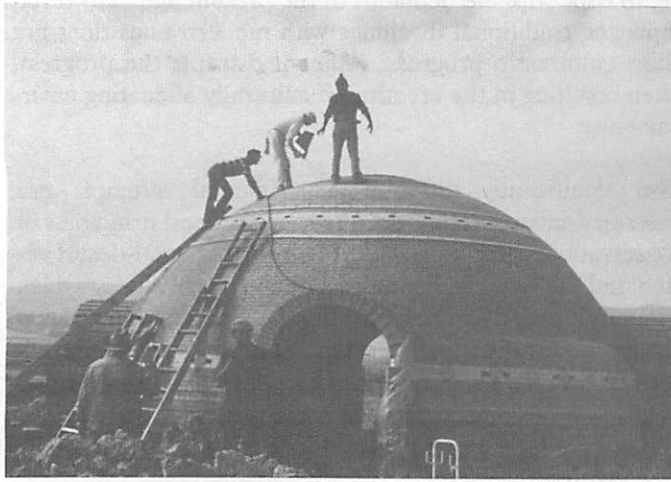
Experimental prototype earthen dome prior to firing in California
