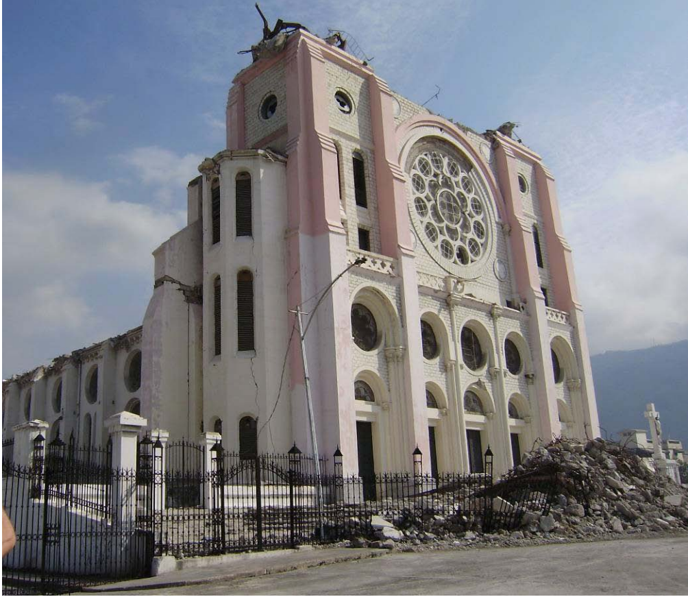
The Cathedral lost the tops of its twin towers and its roof, but most of the interior columns and arches still stand and appear to be repairable
