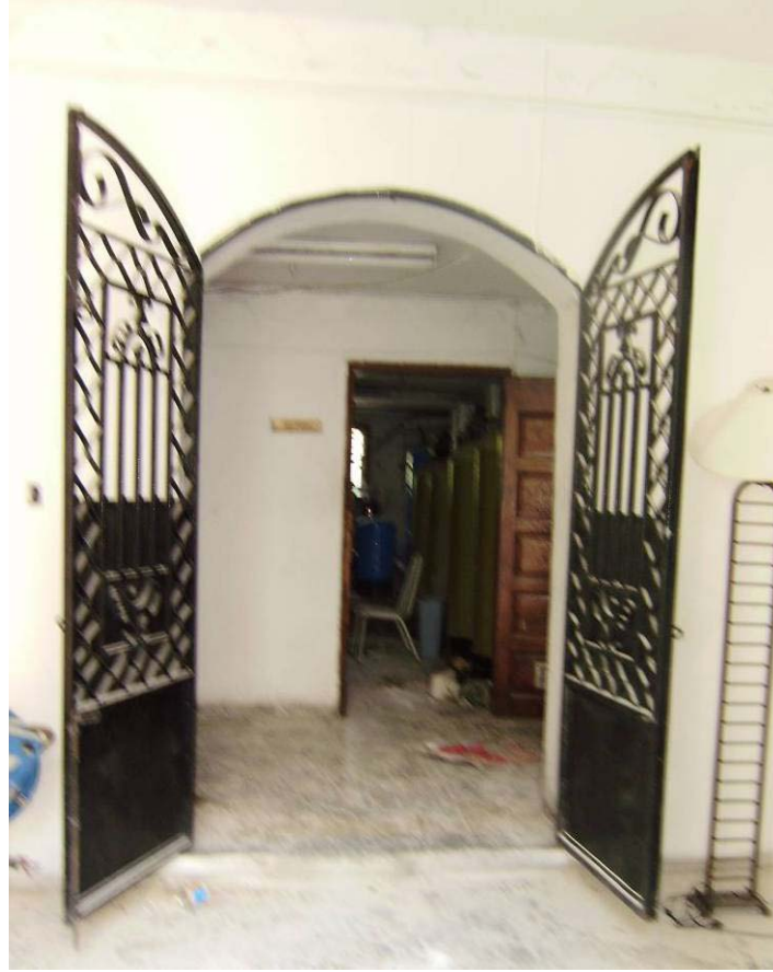
Little or no damage is evident at the Basement Level
